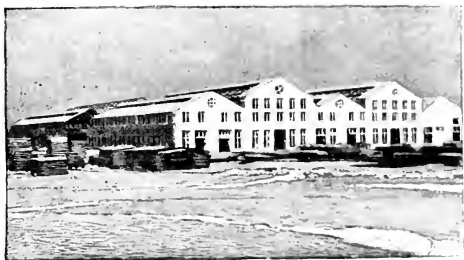
An Electric Company's Plant at Manchester, England.
